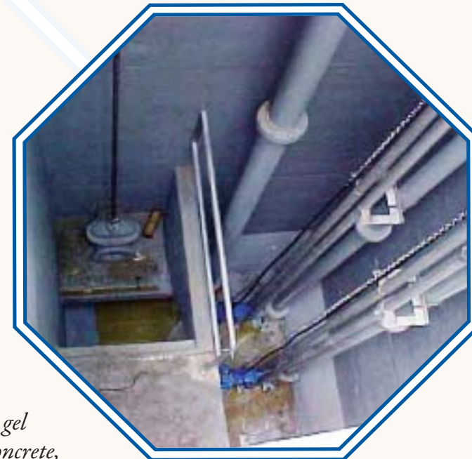
Manhole Rehabilitation USA
