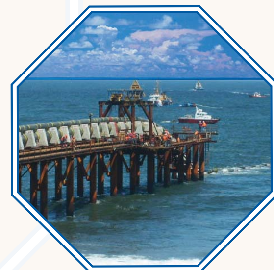
Concrete Weights Santiago, Chile
