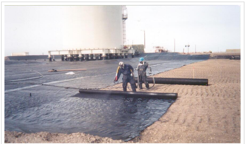
Polycoat Polyeuro® 5502 polyurea applied at 80-100 mils over 8-mil geotextile fabric sheets
